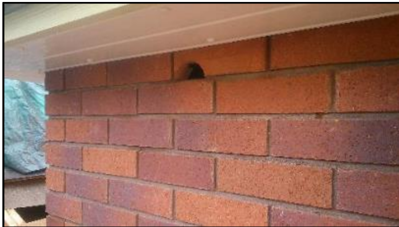
Figure 21: A Swift Brick installed in a newly erected redbrick wall. Photo: www.birdbrickhouses.co.uk .
