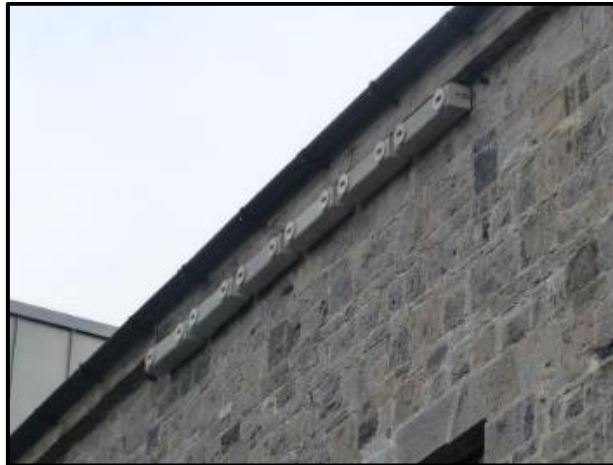
Figure 18: A row of Swift nest boxes installed at Mullingar Courthouse. Photo: Richella Duggan.
