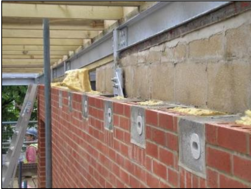
Figure 20: Swift Bricks installed during build phase in Nothing Hill, London.
